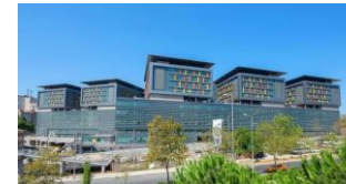
IsDB-funded Okmeydani Training & Research Hospital
