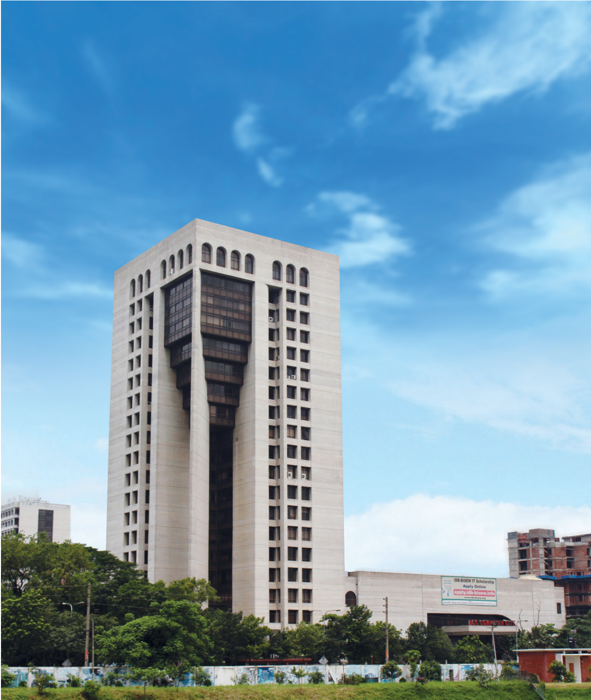
IsDB Bhaban Building, Dhaka, Bangladesh Source: IsDB-BISEW Management Office.
