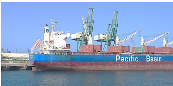
A Rehabilitated Quay, Jorf Lasfar Port
