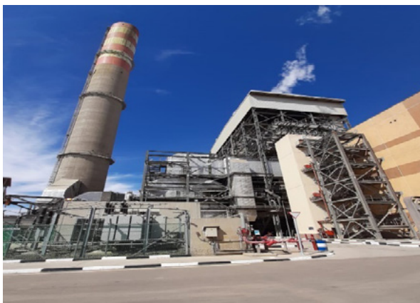
The Al Suez Steam Power Plant
