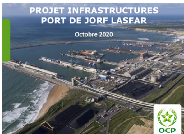
The Jorf Lasfar Port, Aerial View
