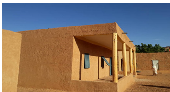
A classroom built by the project
