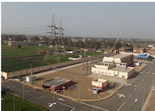
Benha Power Plant Overview
